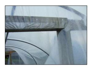
Place the batten underneath the flap of polythene and roll the batten into the polythene, up to the rebate. Nail the batten in place. Note, it is preferable to have a couple of small pleats in the flap of polythene.
