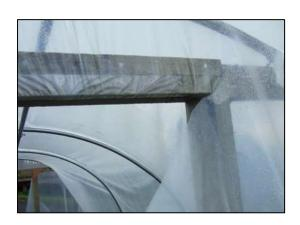
4 Place the batten underneath the flap of polythene and roll the batten into the polythene, up to the rebate. Nail the batten in place. Note, it is preferable to have a couple of small pleats in the flap of polythene.
