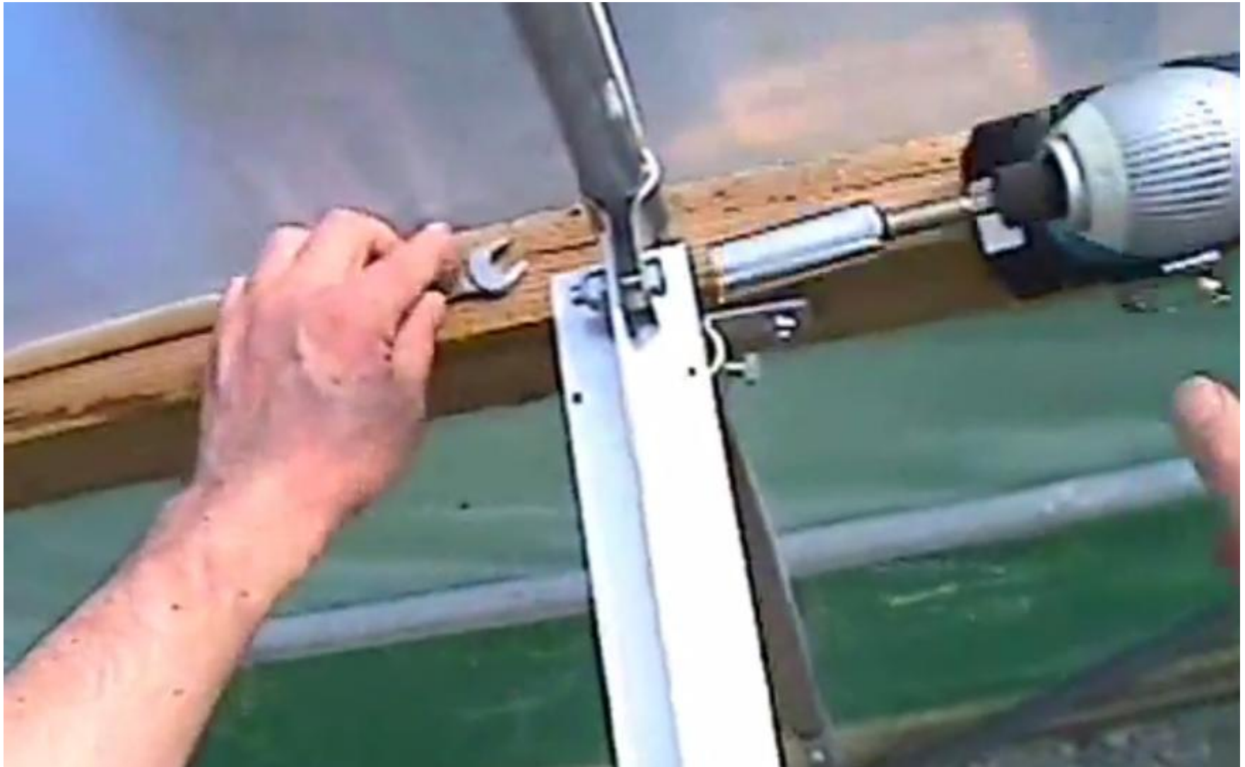
Fis the aluminium arm to the leg of the hoop with the KH 25 fitting
