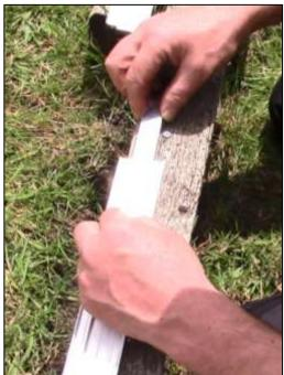
7 Carefully slide the Aluminium Gutter Base sections behind the legs of the hoops, between the polythene cover.
