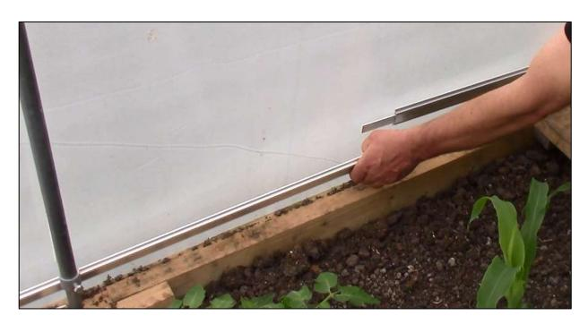
9 Carefully lift the assembled Aluminium Gutter Base up to the correct height, previously marked on the legs of the polytunnel hoops.
