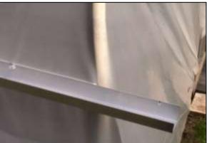
13 Seal over the joints in the Aluminium Gutter with the Gutter Flashing. Peel off the backing and carefully place the Flashing over the joint. Press firmly into place ensuring the flashing seals into the corners of the Aluminium Gutter.
